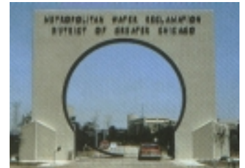
Mainstream Pumping Station entrance
